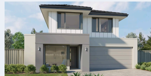
Modern Double Storey
